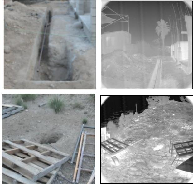
**Figure 5-1.** Top: color and 3-5  $\mu\text{m}$  thermal infrared imagery of a construction trench at JPL, taken at 10 pm. Bottom: color and 3-5  $\mu\text{m}$  thermal infrared imagery of a pothole dug in soil at the same construction site, taken at midnight.
